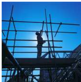
Hard hat missing Fall Protection missing
