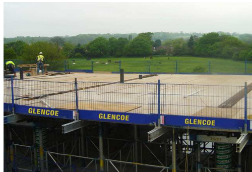
Compliant Side Rails and Toeboard
