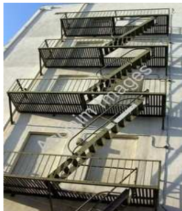
Correct - railings and side guards on all 3 pictures above
